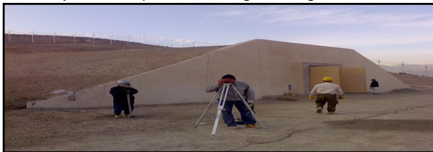
ASP Project at Camp Gambiri Nangarhar Afghanistan
