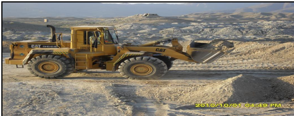
Project at Camp Gambiri Nangarhar Afghanistan by Subcontract
